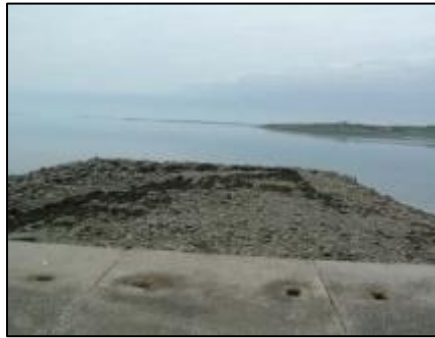
Plate 11 Site CH-11 – from north
