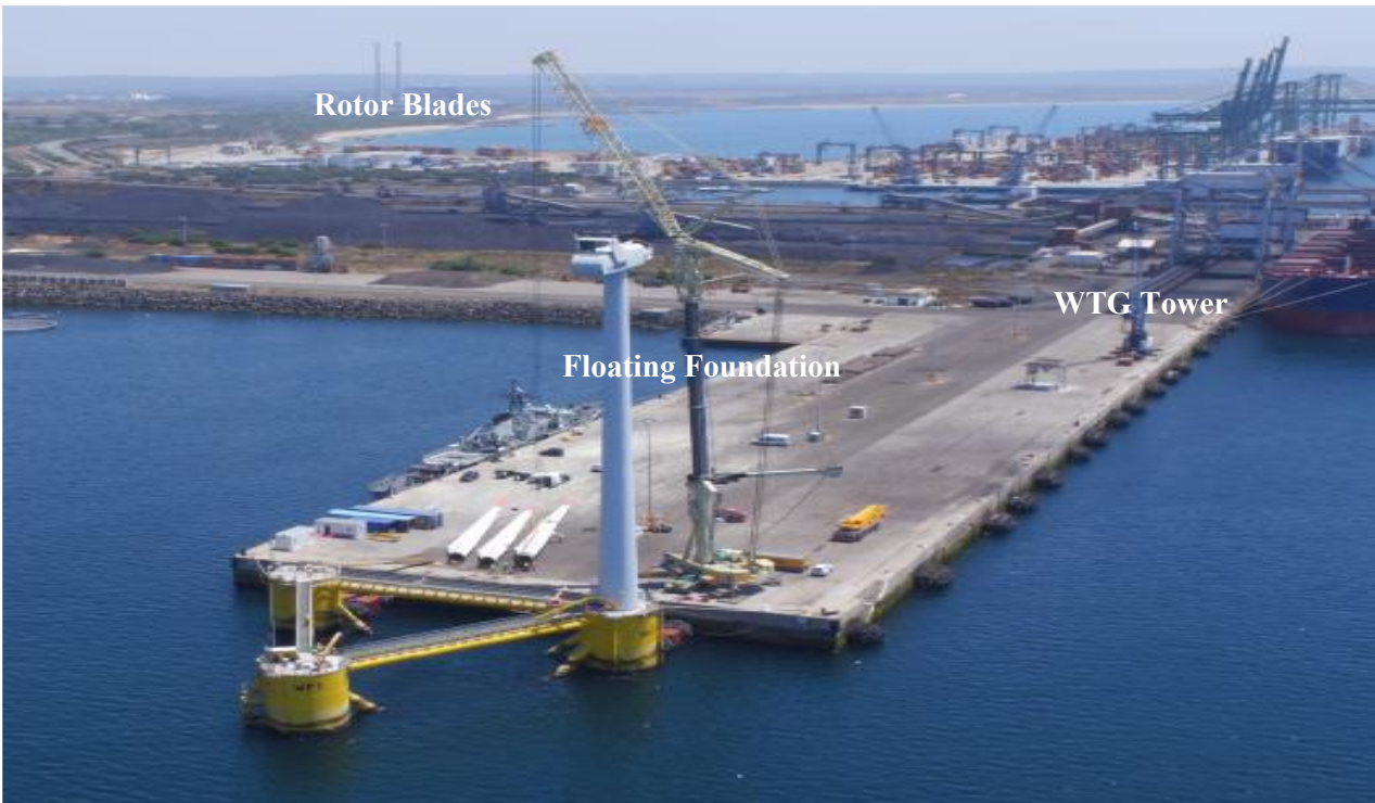
Figure 2.1 Typical construction activity at a quayside construction hub (Source: ESB, 2023)
